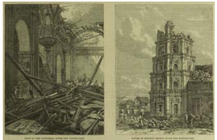
“The Earthquake at Manilla” August 29, 1863
